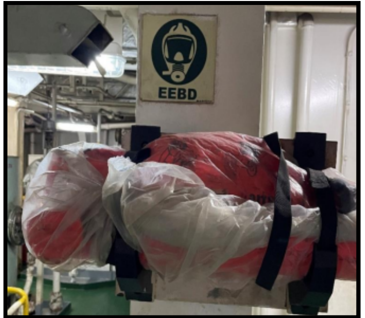
EEBD covered by flammable material (vinyl)
