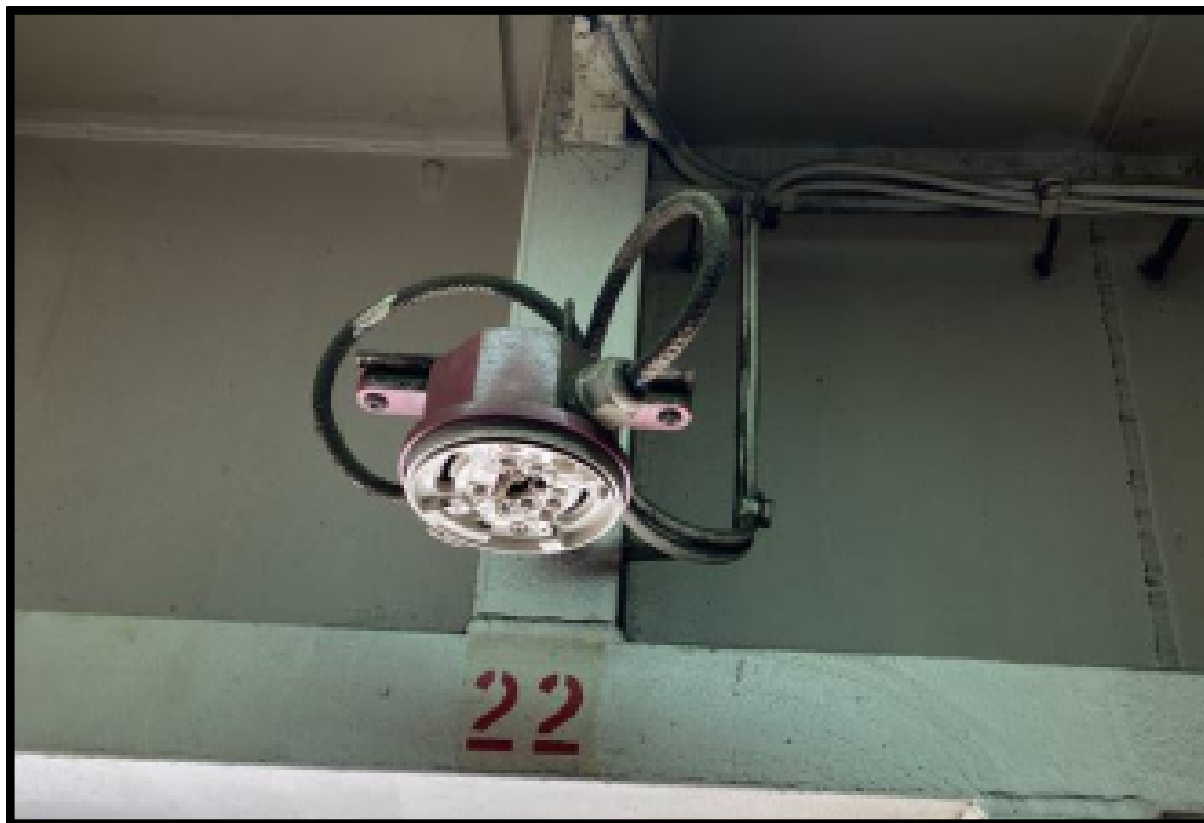
Dismantled fire detector
