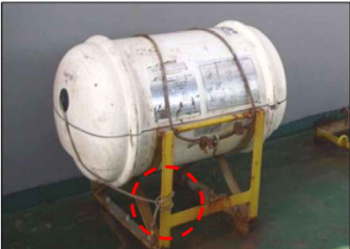
Inappropriate painter securing
