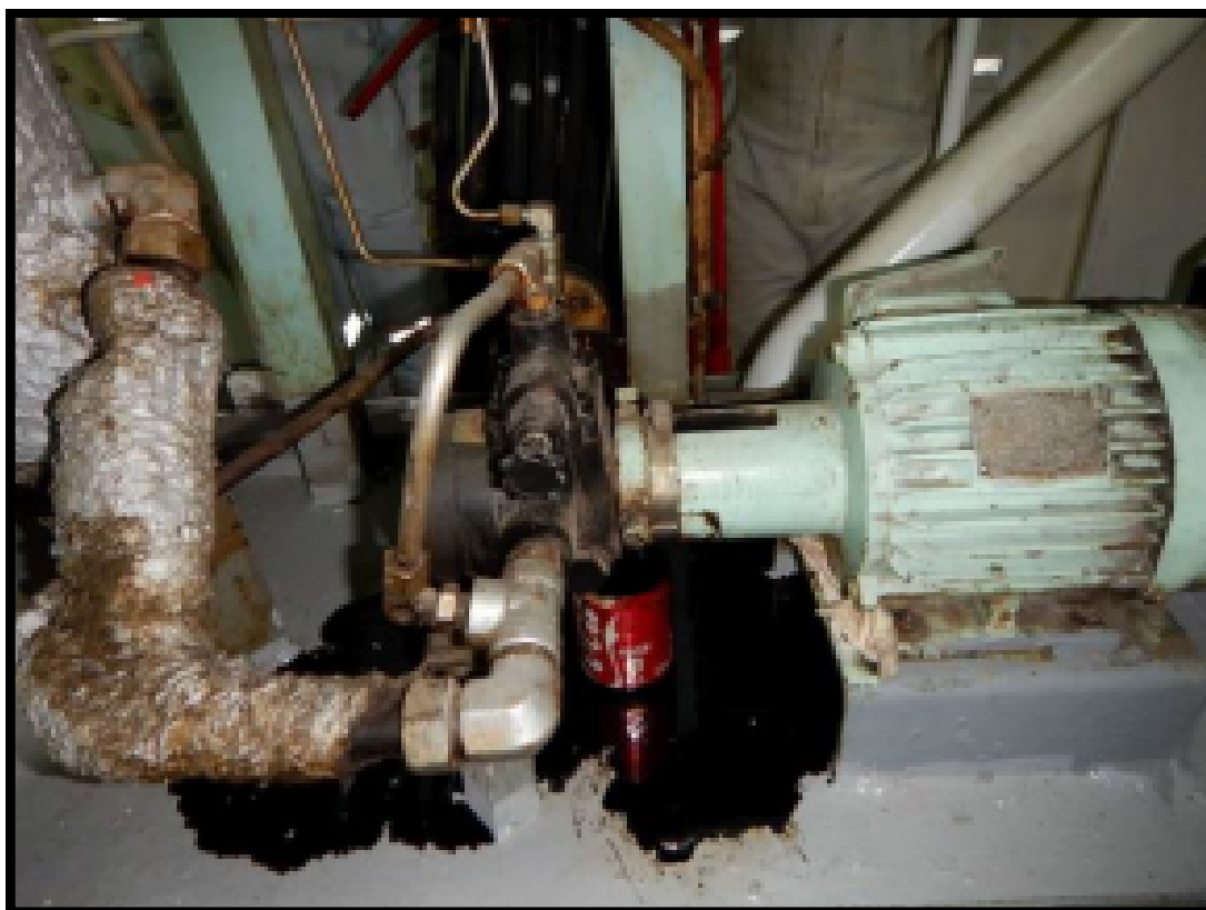
Oil leakage
