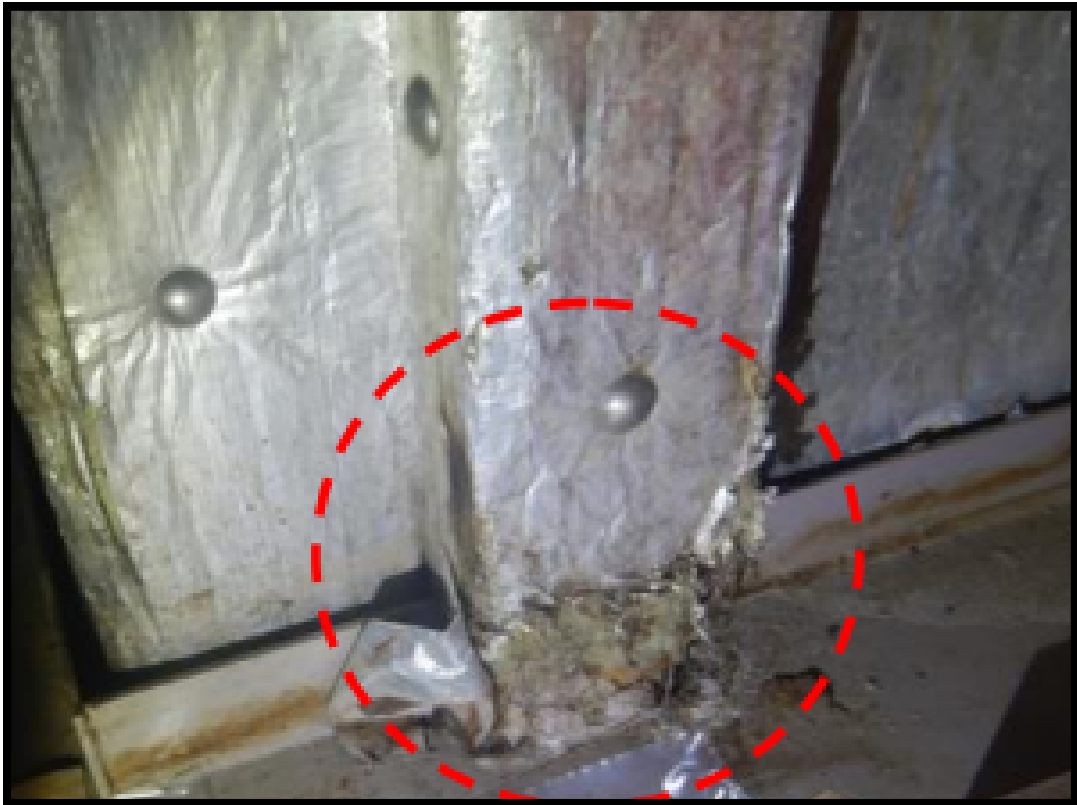
Deteriorated insulation
