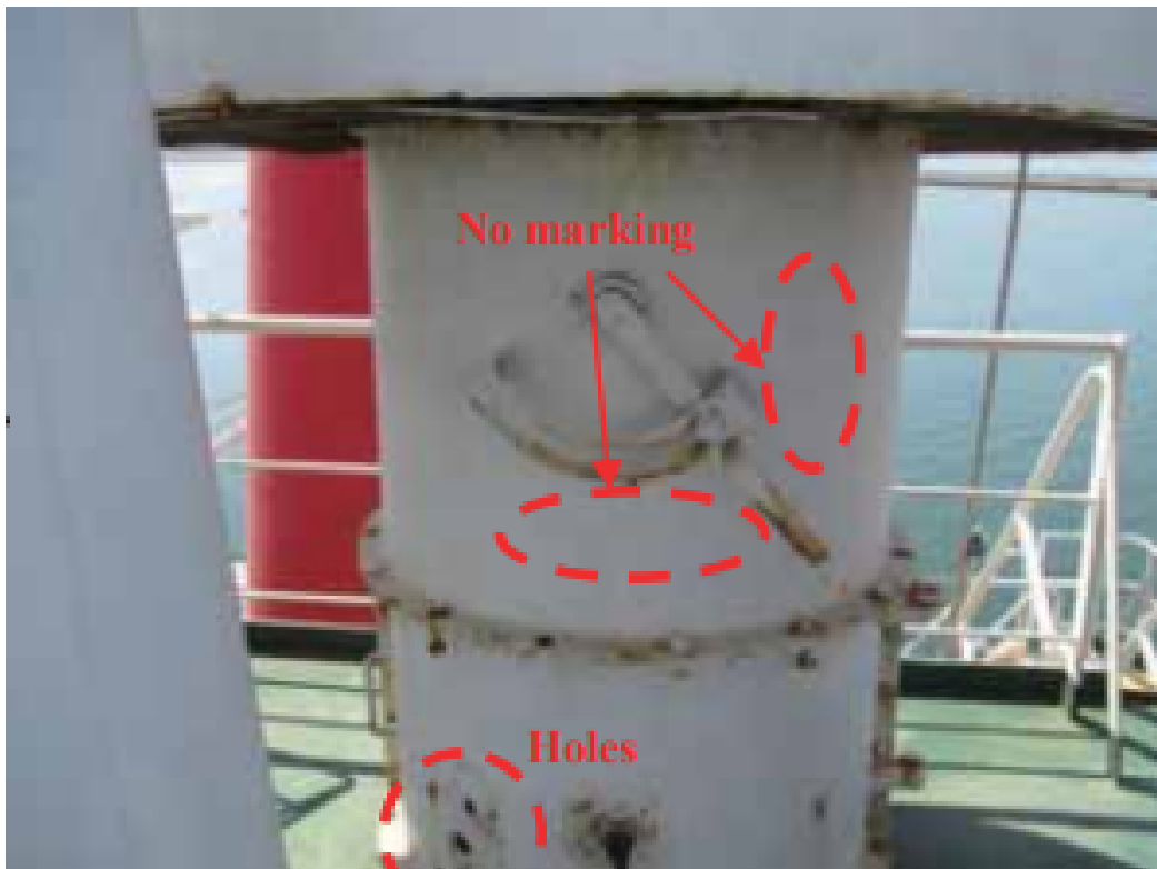
Holes on ventilation trunk and No marking of "Open-Shut" positions
