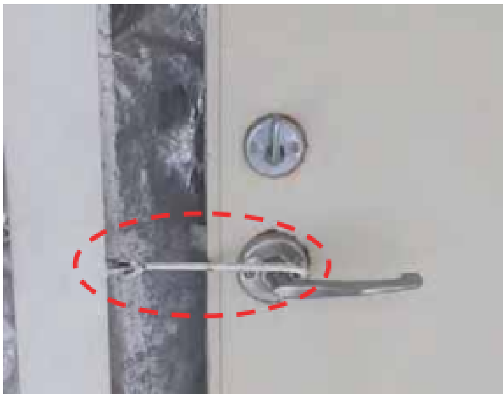
Hold-back hook fitted on self-closing door
