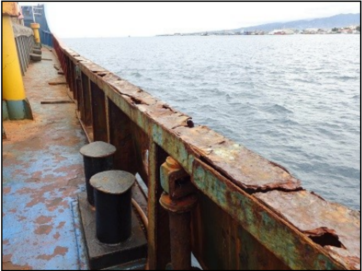
Serious corrosion of the vessel.
