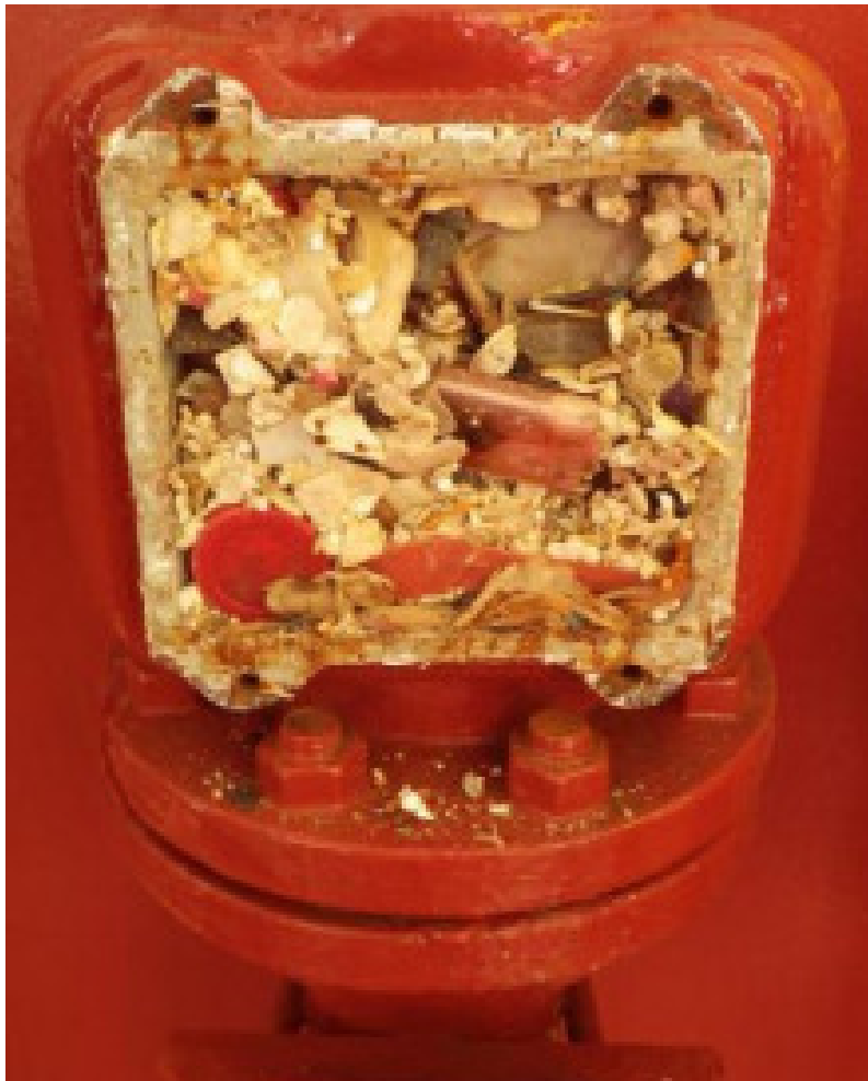
Defective air pipe.
