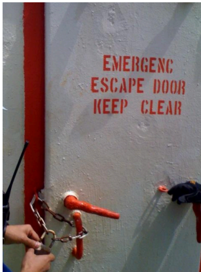
Blocked fuel valve preventing remote actuation
