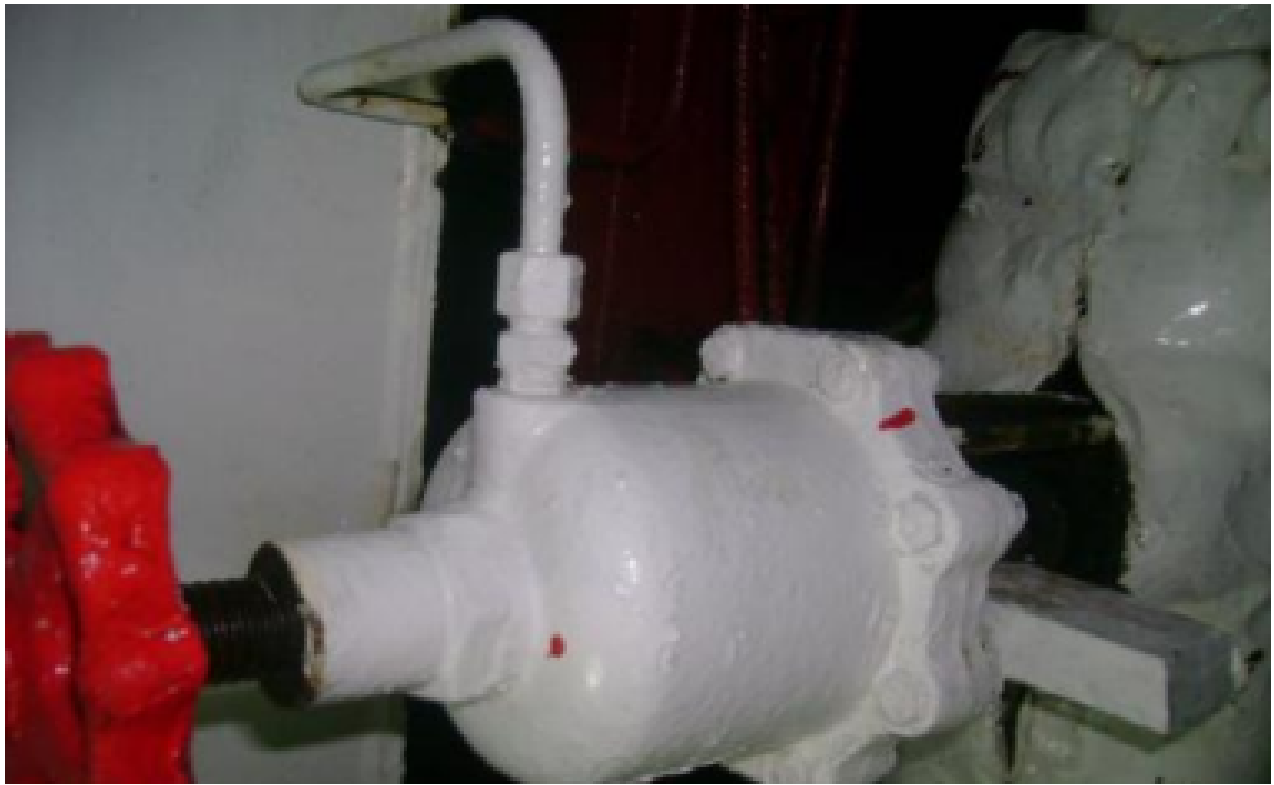
Blocked fuel valve preventing remote actuation
